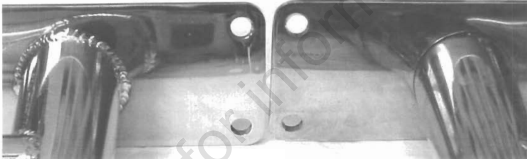
Bracket With Correct Weld Bead
